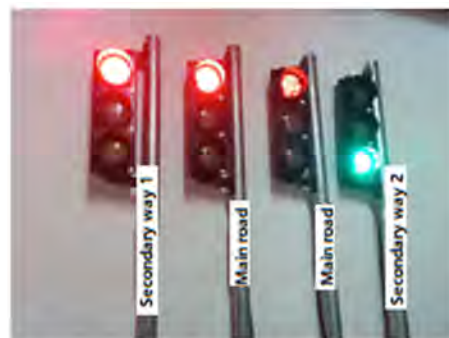
Figure 7. Activated state of lights on secondary way 2.
