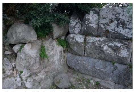
Fig. 8 The curtain wall built with andesite and adjoining tower built with hard limestone, north of the Myndos Gate in Halikarnassos (Taken by author).
