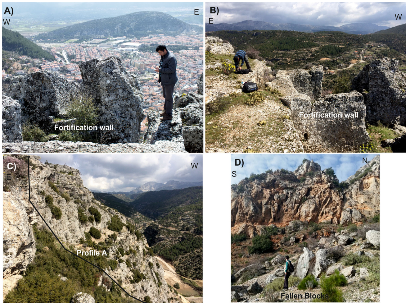
Fig. 4 a The fortification wall block includes stairs. This detached block is just sitting at the edge of cliff (Man for scale 1.73 m). b Another fortification wall block is detached from main hill. Only small earth fill part is located between these two blocks (Bag for scale
