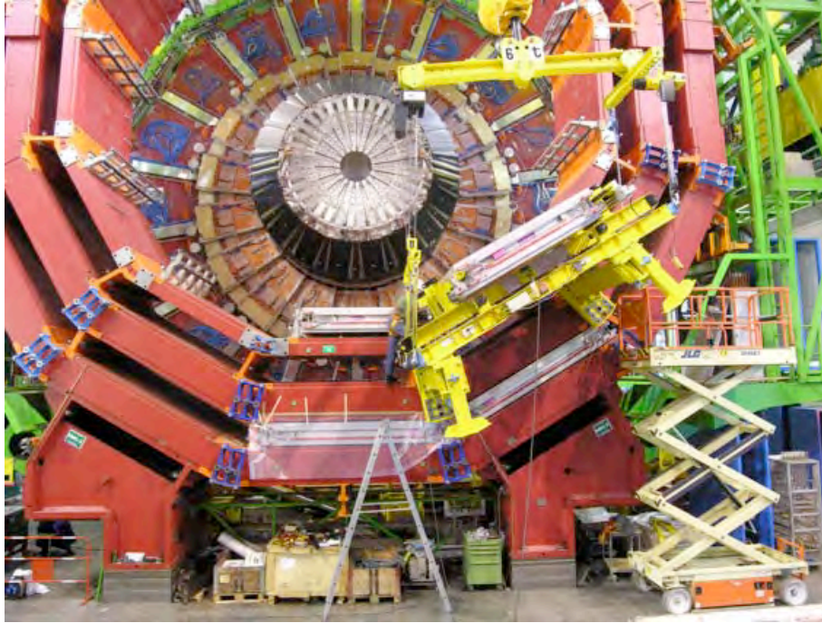
Figure 7.26: Installation of MB1 station on Wheel -2. The yellow frame is the cradle used to insert the chamber in its location inside the iron slot.
