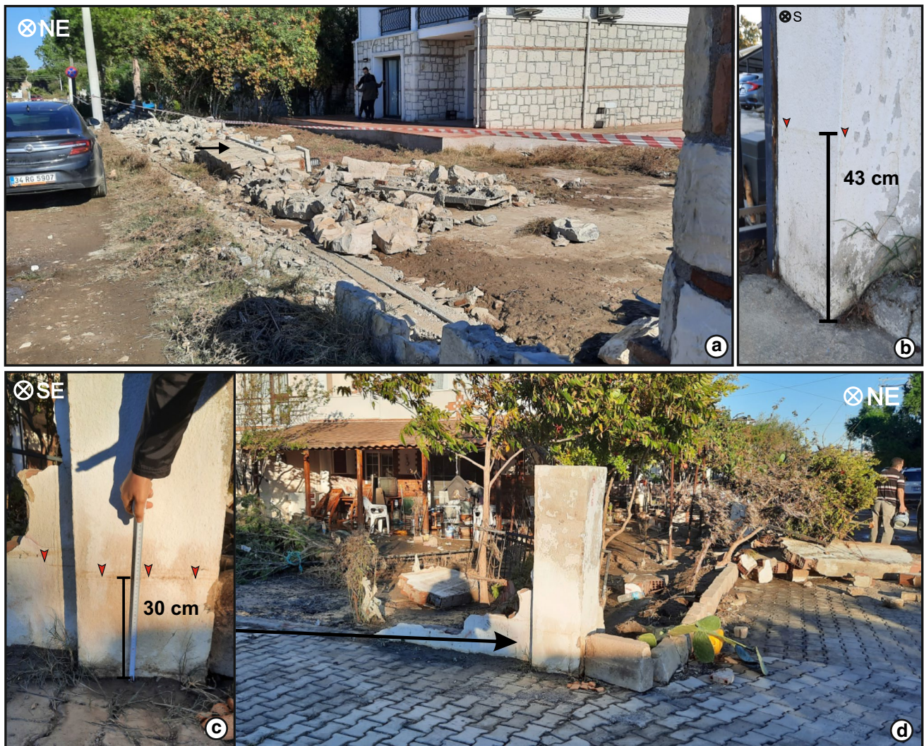
Fig. 8 Approximately N–S-oriented walls collapsed when hit by the tsunami with a flow depth of 30–40 cm at the northern part of Sığacık
