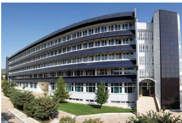
Figure 4 40 kWp BIPV application.
