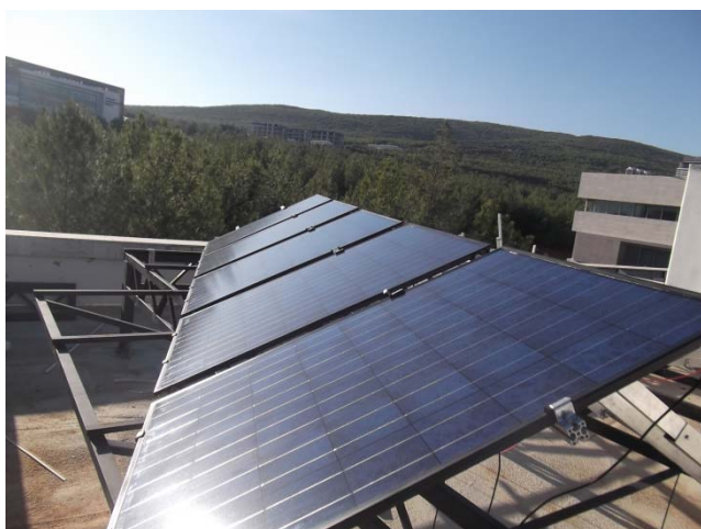
Figure 7 PVT system under test.
