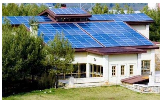
Figure 3 Turkey student cafeteria with 25.6 kWp grid connected BIPV application.
