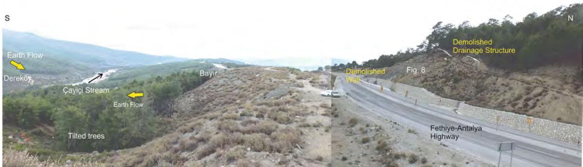
Fig. 9 The earthflow evolved due to toe removal of slope by the Cayıç Stream on both side of its valley
